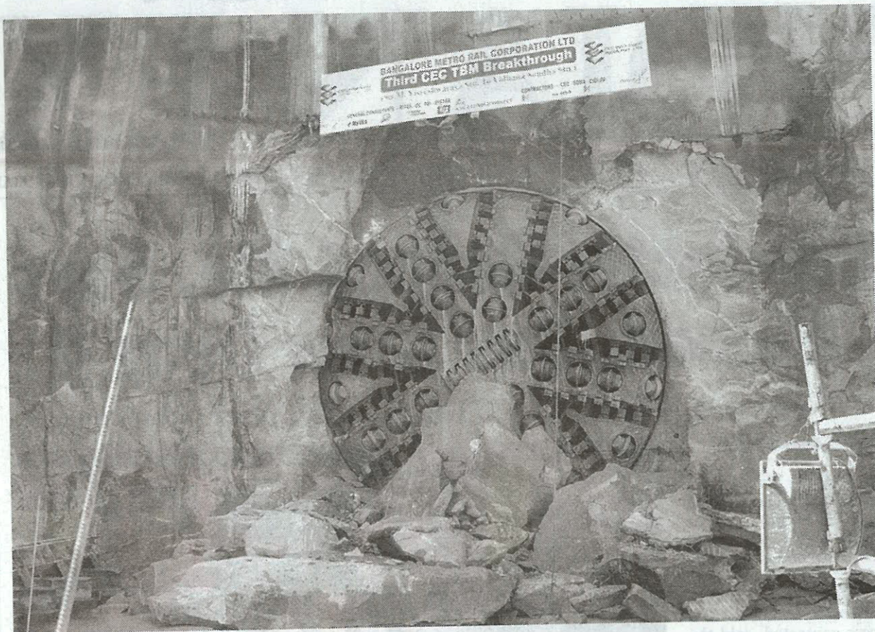
Tunnel Boring Machine Helen in action near Vidhan Soudha
